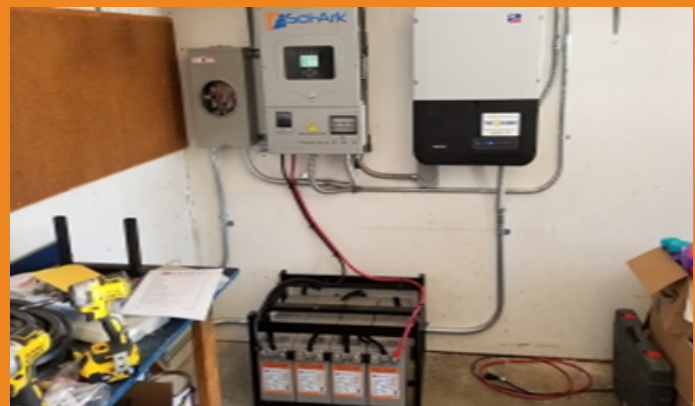
Solar panel installed after site preparation in Masvingo, Zimbabwe.
